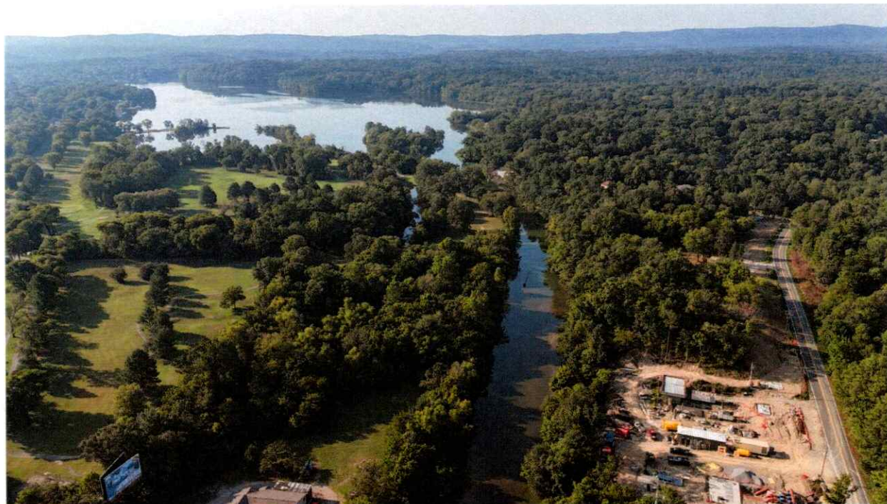
Gulpha Pump Station in Relation to Spencer Bay and Gulpha Creek
