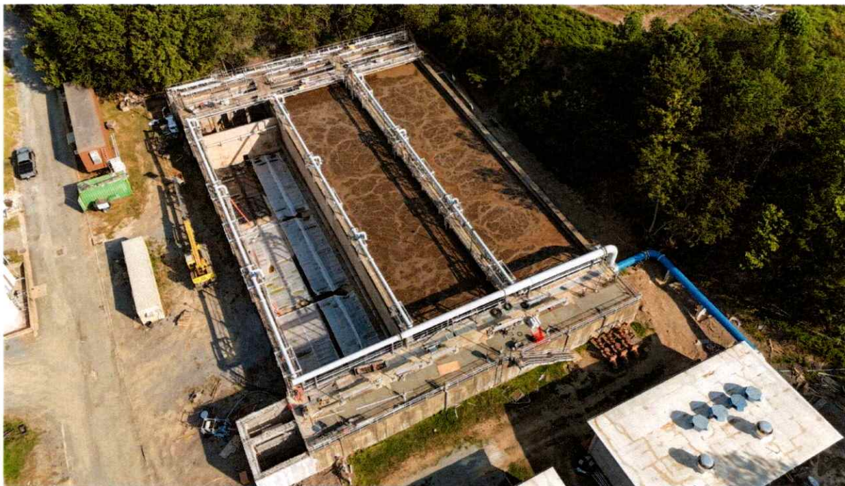
New Diffuser Work in Aeration Basin
