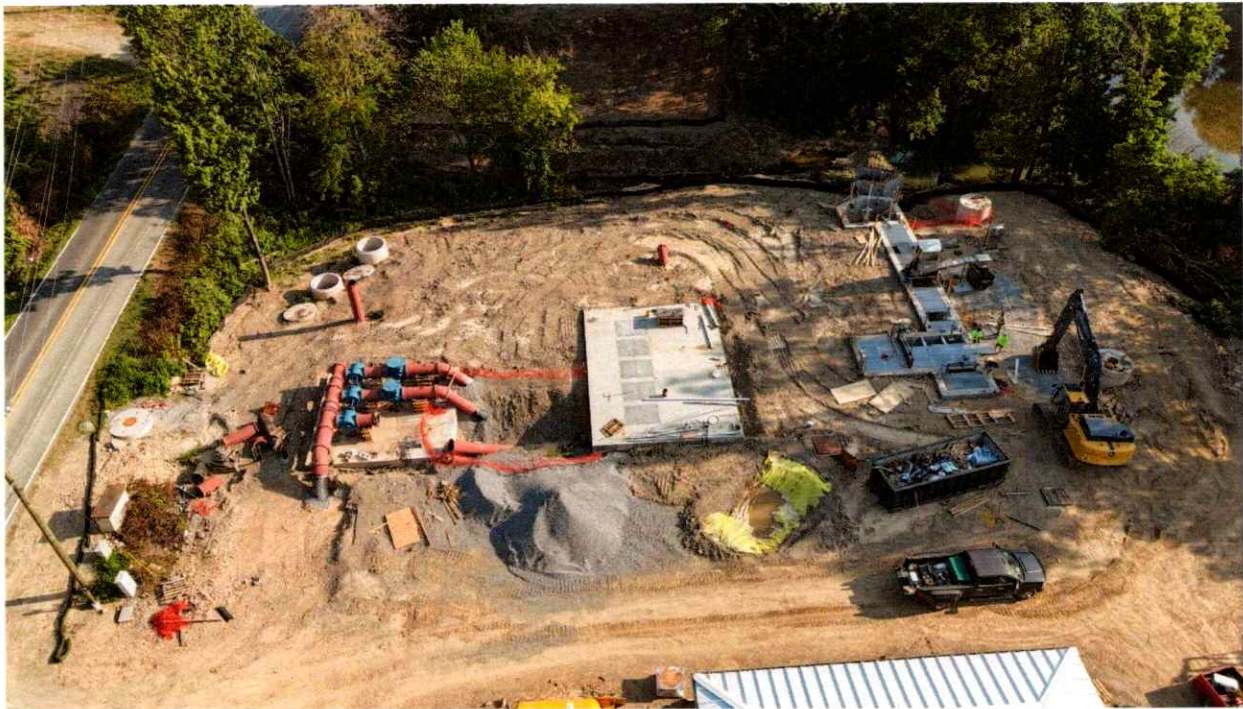
Pump Station Construction in Progress
