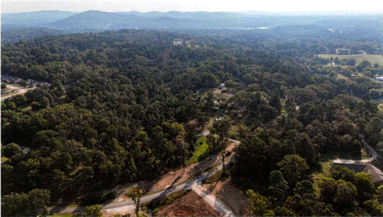
New Line Work From Gulpha Pump Station to Davidson Drive WWTP
