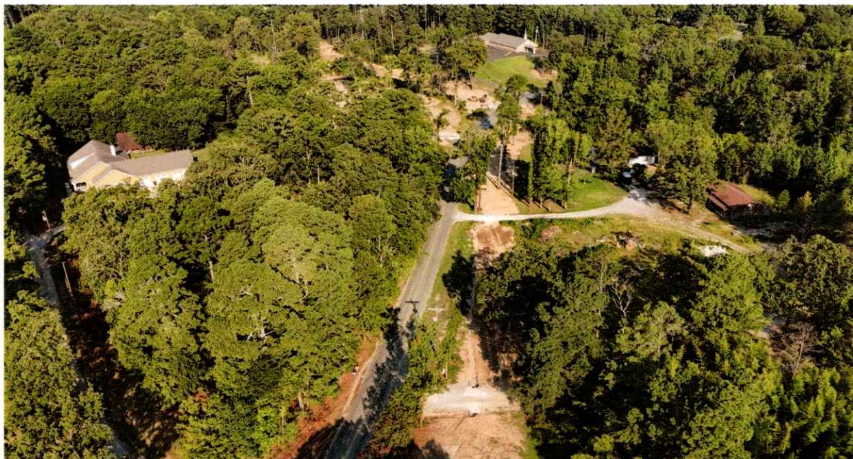
New Line Work From Gulpha Pump Station to Davidson Drive WWTP
